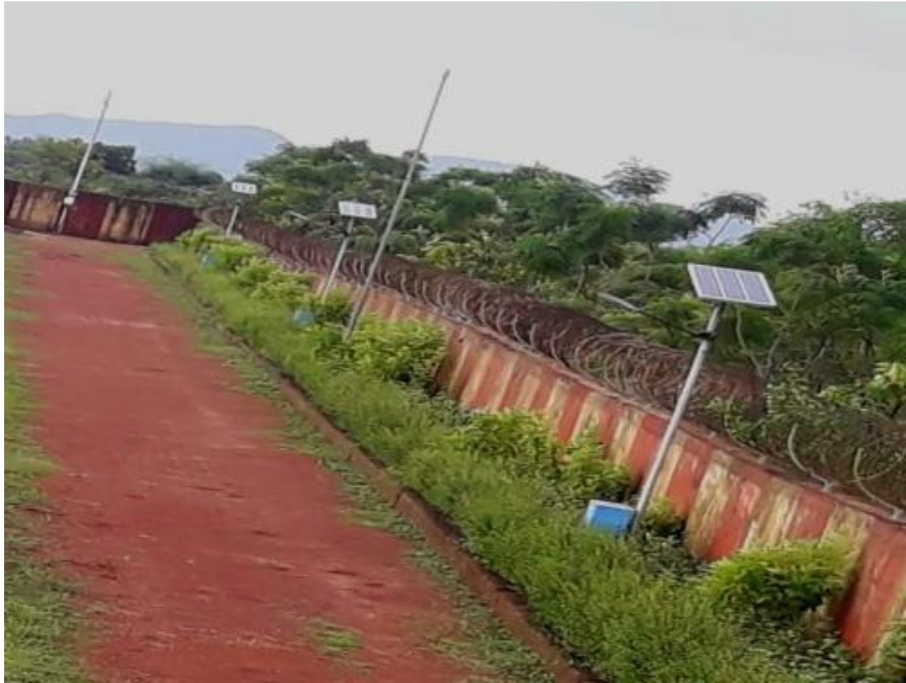
Installation of 125 no.s 50watt Solar Street light for plant area lighting and main road lighting
